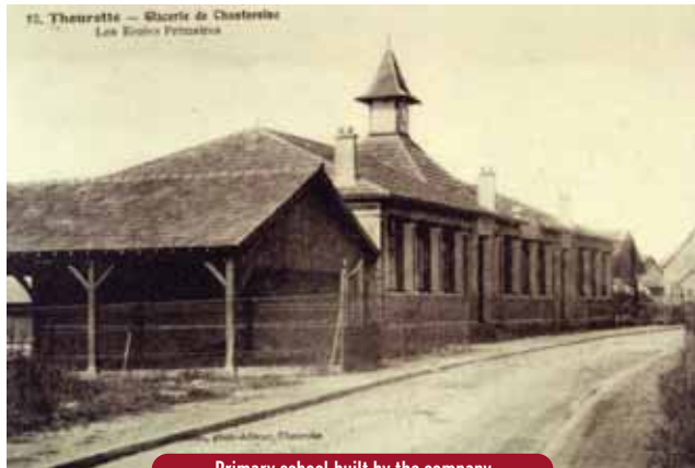
Primary school built by the company
